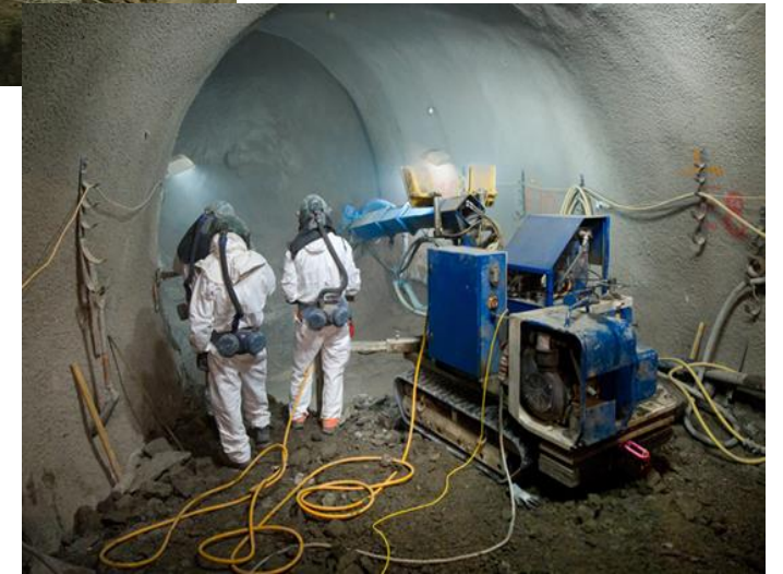
Examples of sprayed concrete lining (SCL) tunnelling
