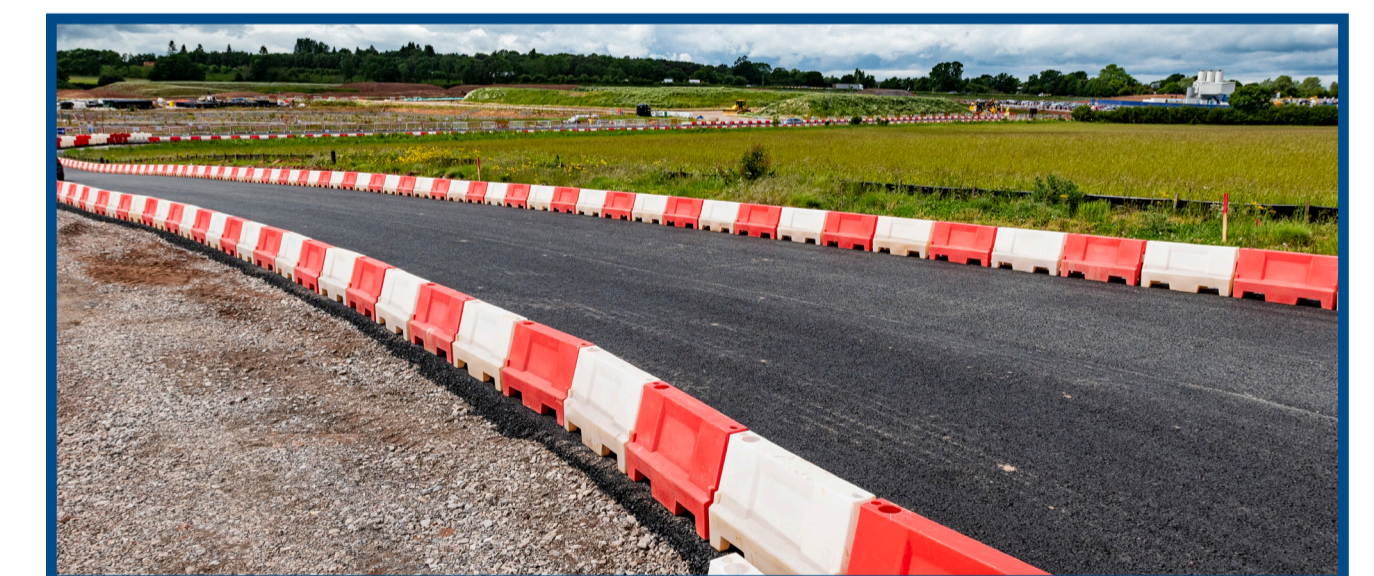
Surfaced haul road in operation at the A46 Main Compound
