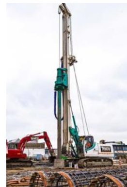
Photo of piling rig
