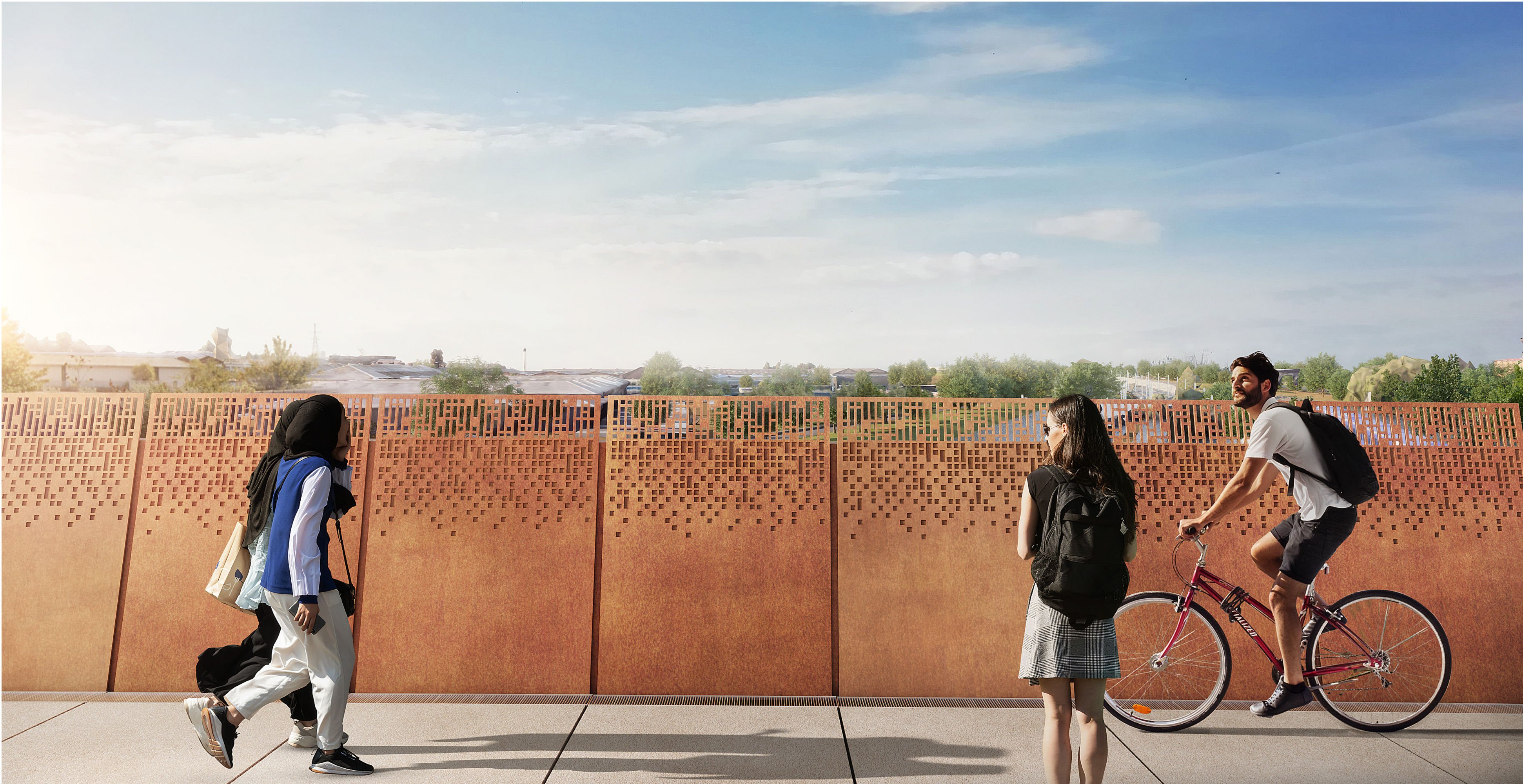
1.8 metre parapet with 0.3 metre high level perforations when over electrified lines
