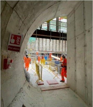
TSS box & tunnel connection
