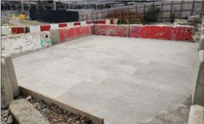
Zone 5 “earth friendly” concrete slab
