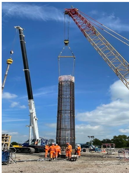
Figure 2: The above image shows our teams installing the first of four piers for the PRA bridge.
