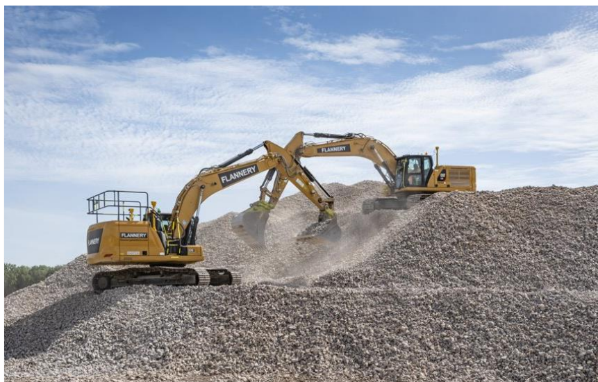
Figure 3: The image presented to the left, shows the aggregate that is unloaded at the PRA site. This aggregate will be used in the construction of many aspects of HS2; such as the construction of the new railway embankment as well as our internal road network.
