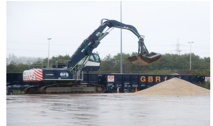
Materials being delivered at the Washwood Heath Depot site
