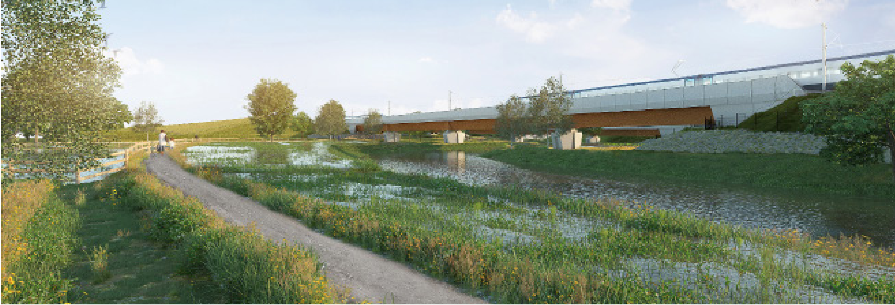
View from public path looking at the River Cole Viaducts with the river partially flooded
