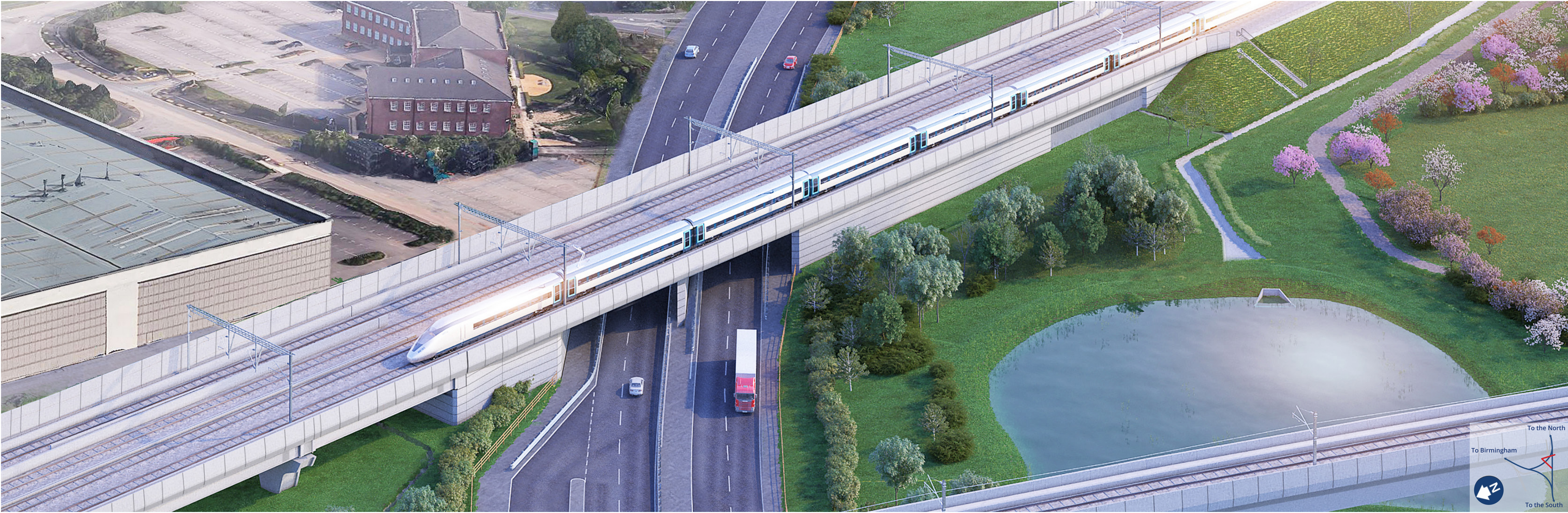
View of the Chattle Hill Structure and Water Orton Viaducts looking south
