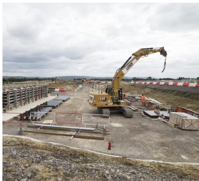
A418 overbridge eastern abutments being constructed
