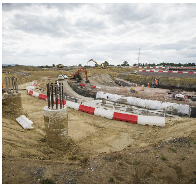
The above image shows the piling foundations for the A418 overbridge.
