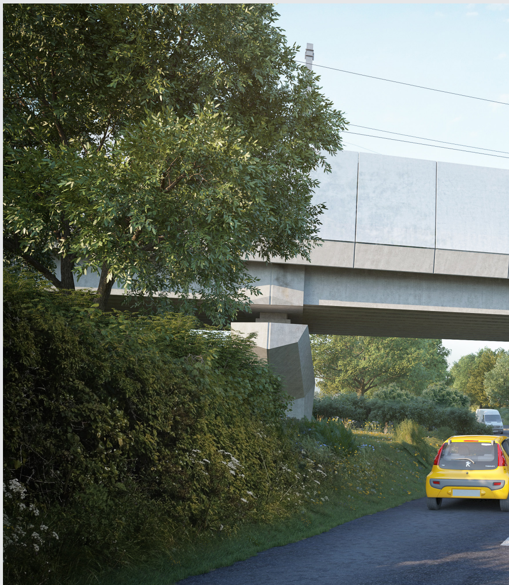
View 3 - from Station Road
