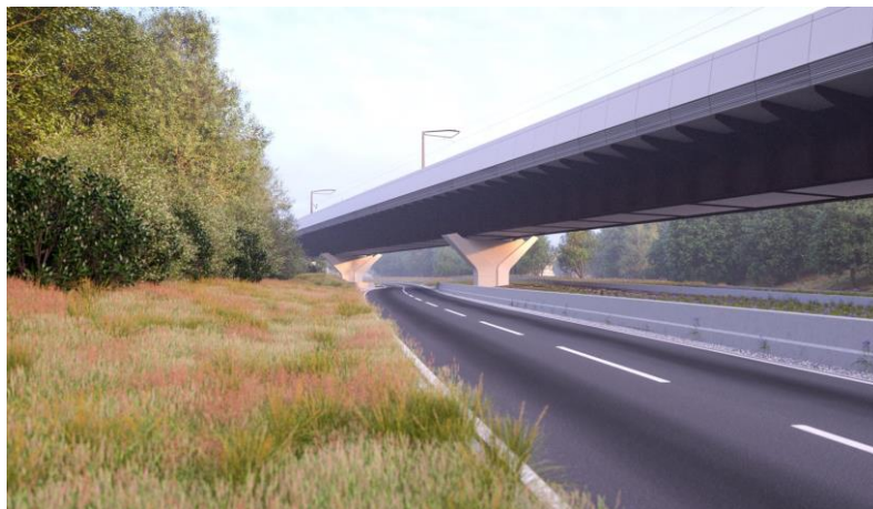
This computer-generated image (CGI) shows the design and span of the Small Dean viaduct and the new alignment for the road.
