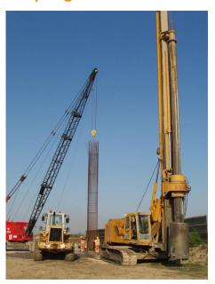
Bored pile is a reinforced concrete pile, which is a commonly used form of foundation that provide support for structures, transferring their load to layers of soil or rock that have sufficient bearing capacity and suitable settlement characteristics.
