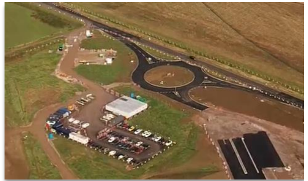
Aerial shot above of the A41 roundabout before completion.
