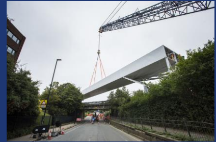
Conveyor crossing installation over Victoria Road and the railway bridge
