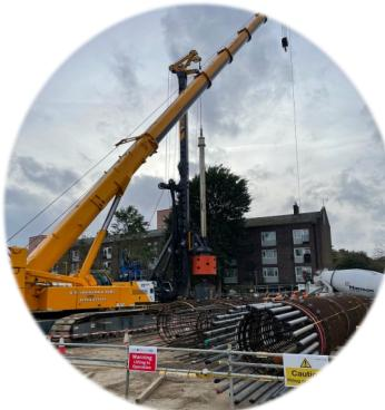
Drilling or boring this way is far quieter than hammering piles into the ground. A crane then places a steel cage into the hole and concrete is poured in to fill the hole. Once the concrete pour is started, it must be finished the same day to ensure the pile is constructed safely and allowed to set overnight.
