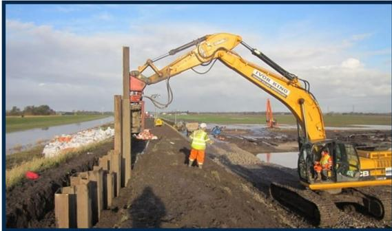
Vibratory piling is a method of installing sheet piles using an excavator attachment known as a Movax. Whilst we always aim to use the least disruptive method of piling where possible, which is pressed sheet piling, there are locations where we have to use vibratory sheet piling. We need to use vibratory sheet piling in the Euston cavern worksite located in the cutting. This is because the space between the live railway and our worksite is too small to accommodate the
