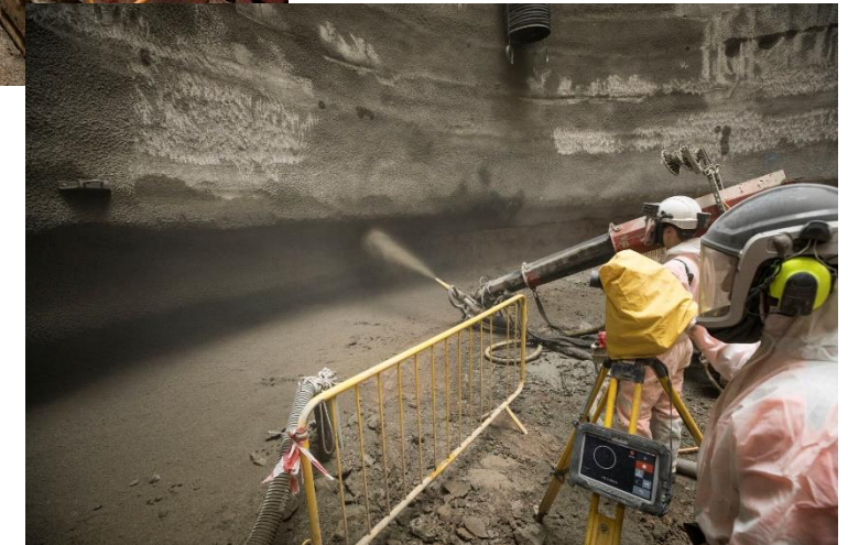
Examples of sprayed concrete lining (SCL) tunnelling
