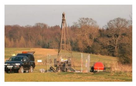
Concrete 'Test Piles' will also be formed in one location near to the works compound. These are concrete foundations formed by excavating a small diameter deep holes and filling it with concrete. Five piles will be formed that are 1.5 metres in diameter and around 40 metres deep.
