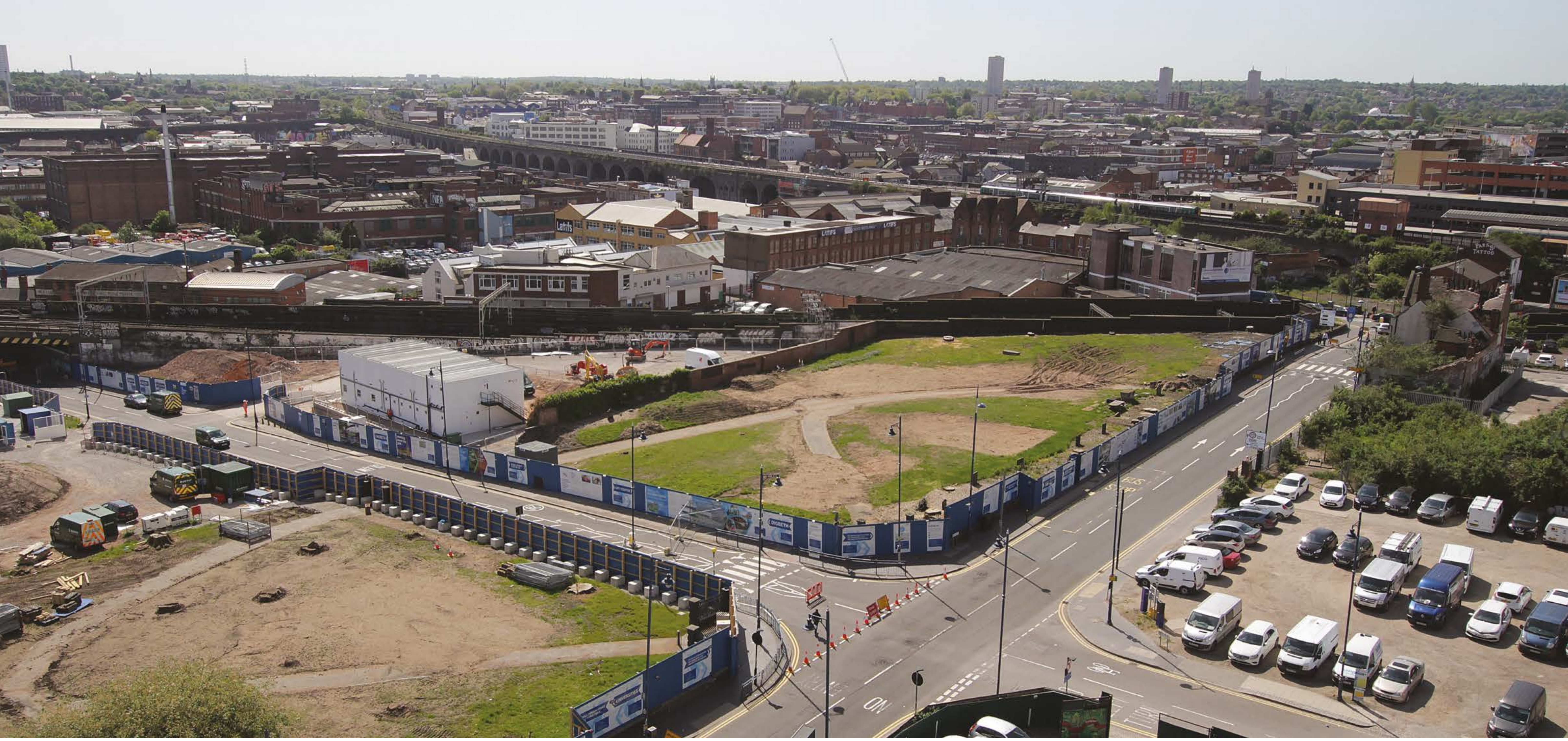
Park Street Gardens construction compound for Curzon Street station, Birmingham
